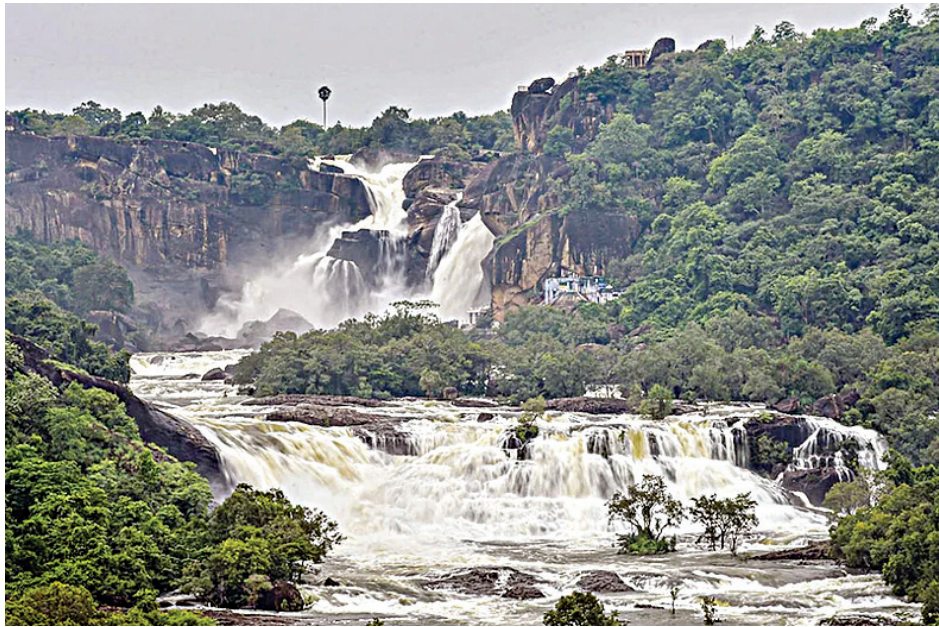
A view of water gushing down hills after the shutters of Papanasam dam were opened to discharge surplus water, following continuous rainfall, in Tirunelveli, Tamil Nadu.
